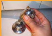
C. Pulling off the bit which turns
