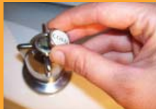
B. Taking the little disc off the top of the tap
