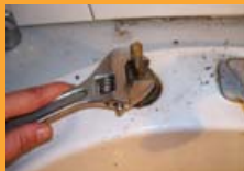
E. Unscrewing the tap body
